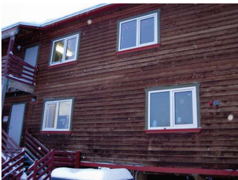
Exterior Windows in Good Condition
