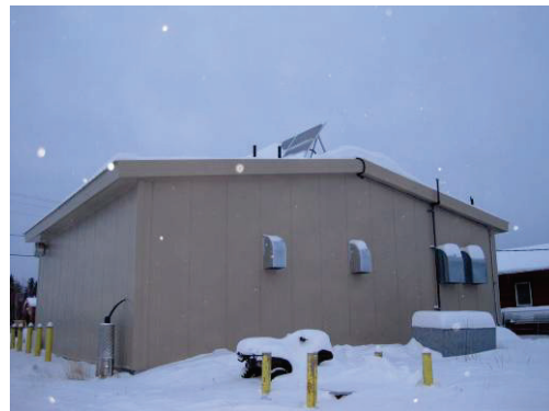
Building Exterior – Solar Panels on Roof
